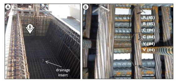
Figure 5-9: (A) End-region reinforcing in Beam 5; (B) six side-by-side bars (two #5s and four #4s) bundled together in the end block of Beam 5.
